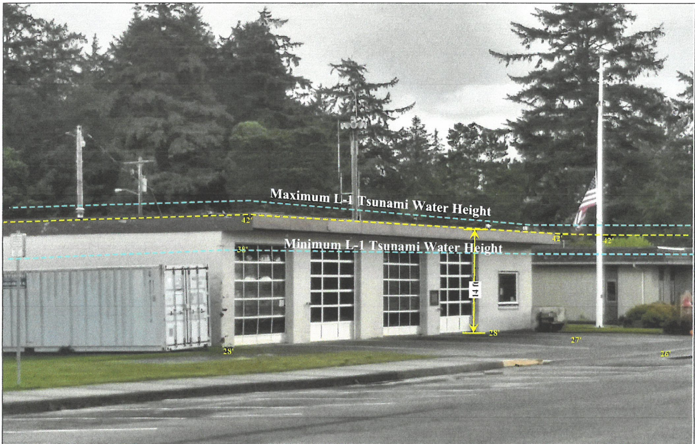
Figure 4: Tsunami for the L-1 Scenario is modeled to flood to 40 to 42 ft, or to about the roof of the existing fire station. For the M-1 Scenario, water would flood to about 30 ft, or barely into the station. There is some variation in the water height here, because one source of information (TIM Clat 08) is for flooding at E Street, and another shows water depth for this site as greater than 10 ft and less than 20 ft (Priest and others (2015)).
