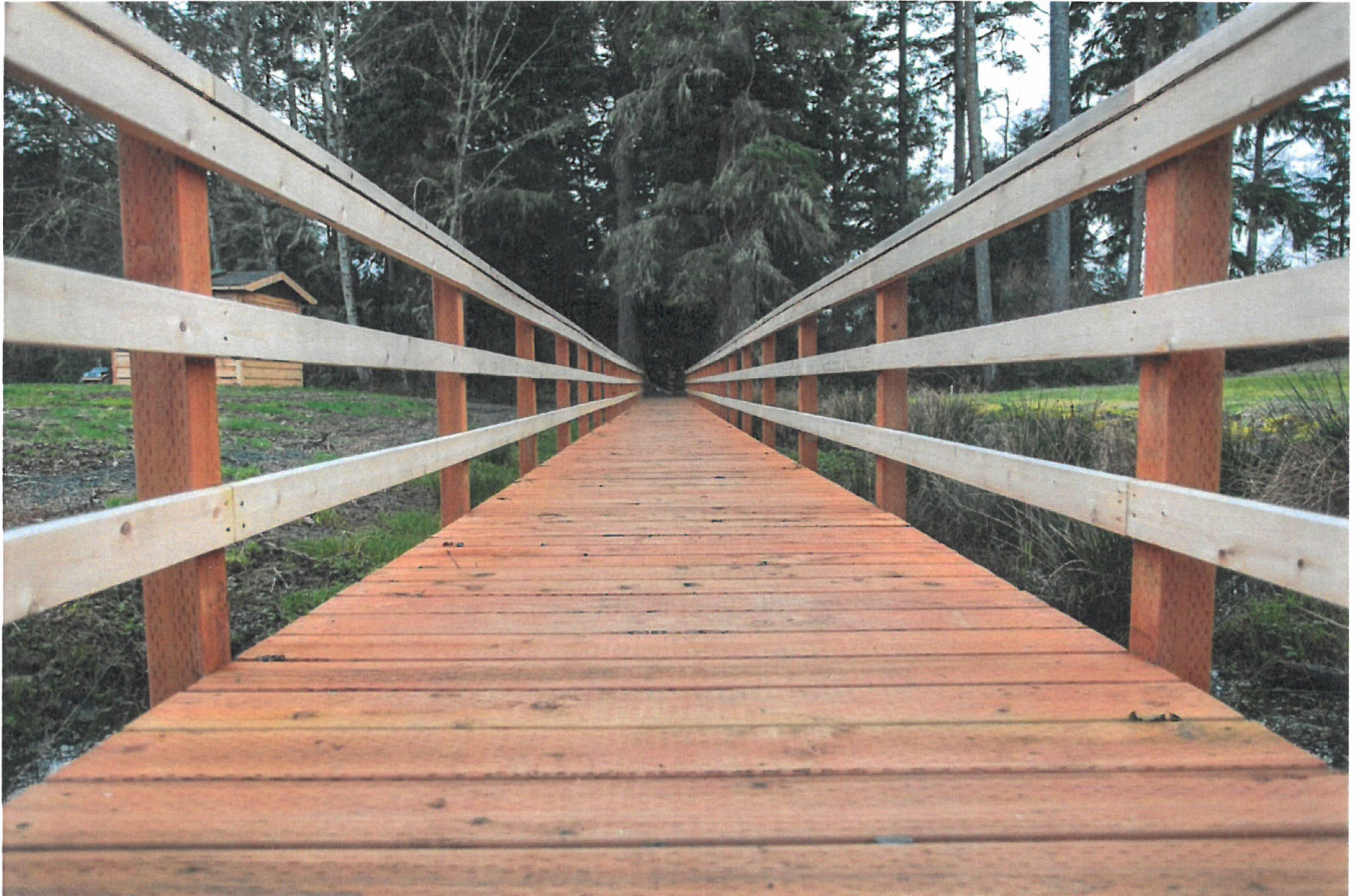
Ridge Path Bridge
