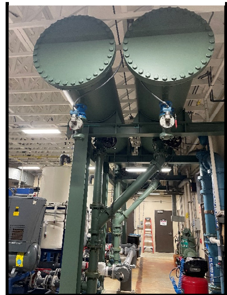
FIGURE 2-6: RAW WATER STORAGE
