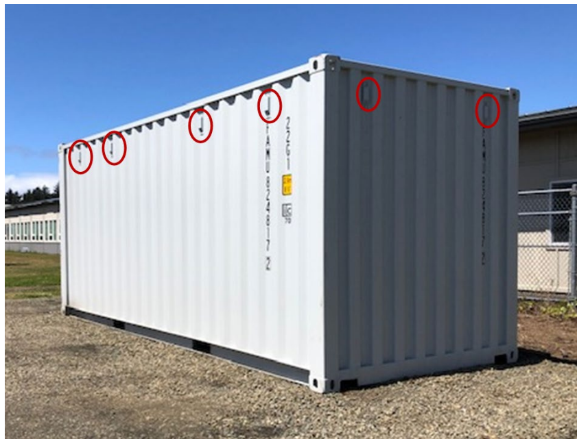
Figure 18: Shipping Container with 12 Built-in Vents Photo courtesy of Susan Graves
