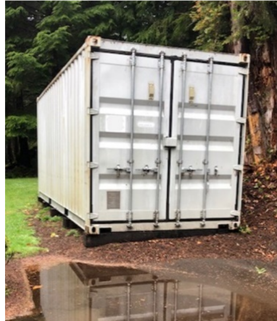
Figure 13: Shipping Container on Five Railroad Ties for Leveling and to Protect from Water Pooling Photo courtesy of Susan Graves
