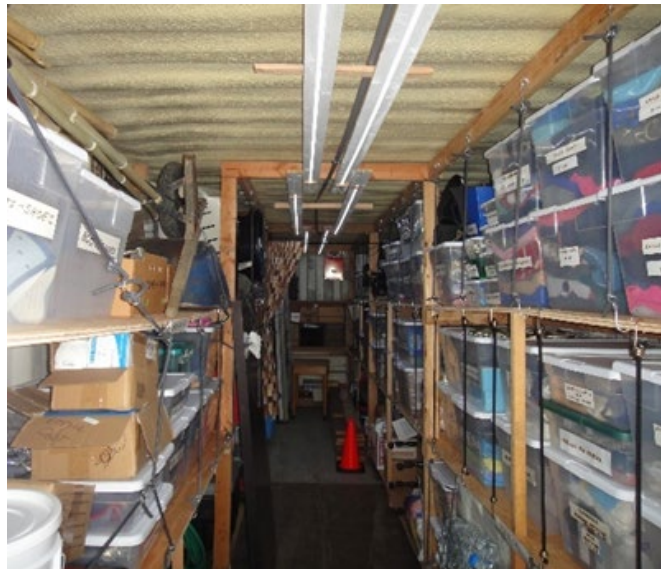
Figure 29: Custom Shelving with Stabilizers
