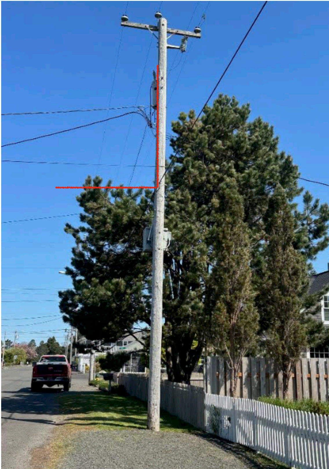
Mandatory clearance window for power lines
